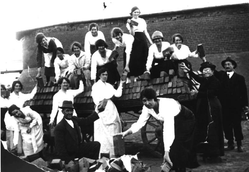
1920, Lucas Girls load bricks for onto horse-drawn carriage for construction of Arch of Victory. Source: Max Harris Photography Collection
